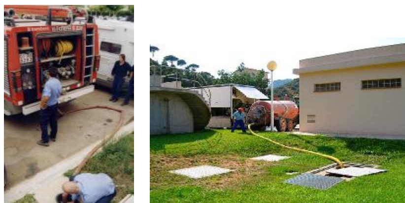
Figure 8. Two images of non-potable uses in municipalities on the northern Costa Brava. Left: Firemen charging at the hydrant of the WWTP in Port de la Selva, summer 2003. Right: Cistern loading reclaimed water from the storage tank of the WWTP in Portbou, for use on the construction of the new road, 30th June 2005.
