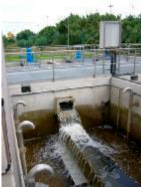
Figures 1 - 3. Pictures of the water reclamation process at Blanes and the reclaimed water produced: on the left, details of the filters; in the centre, disinfection equipment with ultraviolet light; and, on the right, picture of the point where the reclaimed water comes out in the bank of the Tordera.
